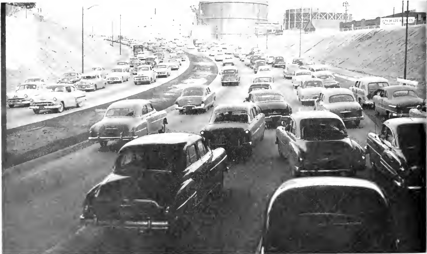
This is a sample of the traffic on the Santa Ana Freeway in downtown Los Angeles, just west of the Aliso Street Bridge over the Los Angeles River, which must be carried with a minimum of delay through two major construction projects—the widening of the bridge and, just beyond it, the adding of a new ramp to the Santa Ana-San Bernardino Freeway interchange.
